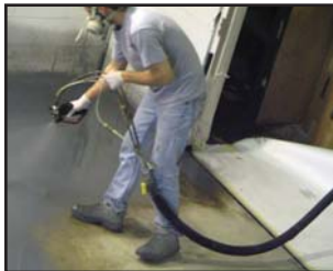
Protective Coating - Concrete Floor.
